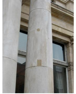
The portico pillars showing the repairs made after the building was damaged by gun fire when it taken over by anti-treaty forces in March 1922 to provide accommodation for refugees fleeing from sectarian attacks in Belfast
