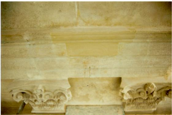
The Remers mortar is applied matching the colour and texture of the stone
