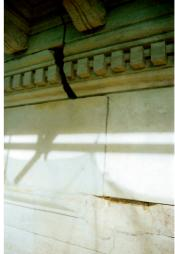
Bursting caused to the decorative masonry at the base of the pediment and just below it due to the rusting of iron cramps
