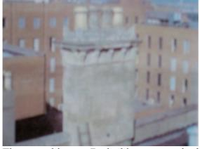
The west chimney. Both chimneys required Stabilising and re-pointing works
