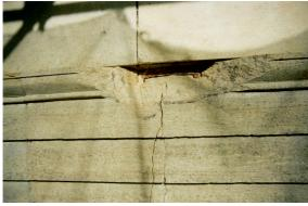
Before repair the stone is cleaned and raked out
