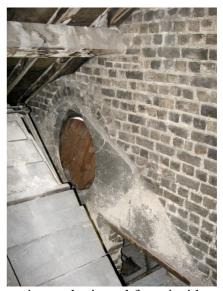
The rear of the west parapet showing the older reconstruction and, viewed from inside, the roof timbers showing the effects of a significant ingress of water a long time ago
