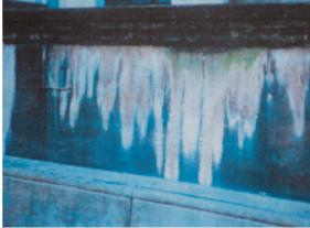
The façade at street level showing the signs of serious staining and caused by urban pollution, and washing with acid rain
