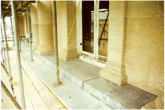
The flashing between the second and third storey was completely replaced
