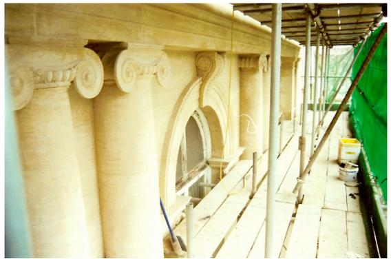
Cleaning in progress at the top of the second storey. The stones original colour has been revealed
