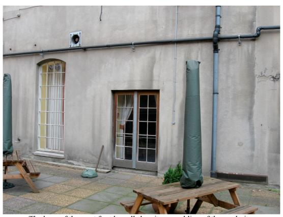
The base of the west façade wall showing crumbling of the rendering
