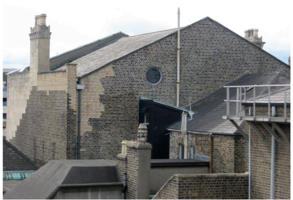
The rebuilt parapet at the rear of the front roof. The intervention is denoted by the use of machined yellow brick
